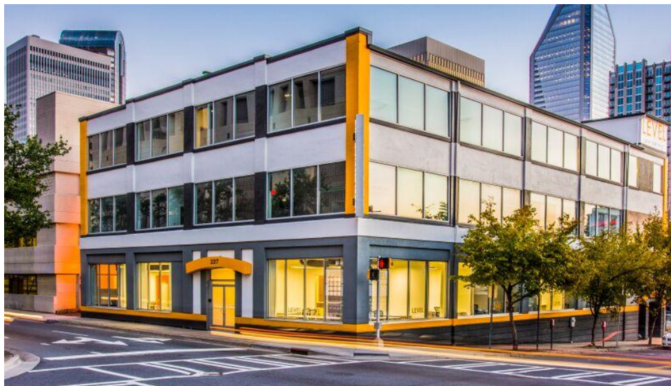
Exterior of new Level Office at 227 West 4th Street.
